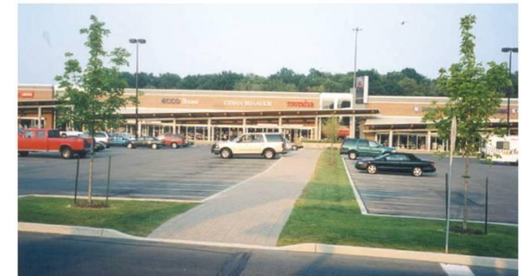
A walkway provides a safe pedestrian connection through a parking lot
