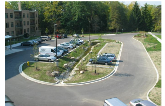
Bioswale incorporated into landscaped area within parking. Curb cuts allow water to enter into bioswale area
