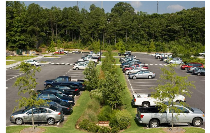
Paved areas are sloped towards vegetative stormwater control area
