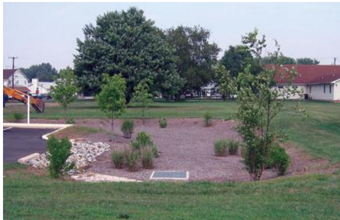
Bio-retention areas can be situated adjacent to parking areas to collect stormwater runoff and encourage infiltration
