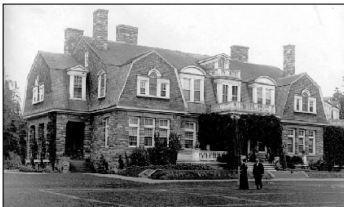
Figure 31: Clergue's home on Moffley Hill - Montfermier (SSMPL 2008)
